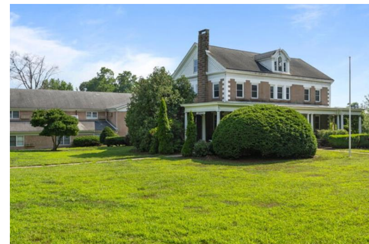
745 Burnside Avenue (Stone Academy)
