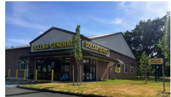
The new Dollar General development on Silver Lane was completed in 2017
