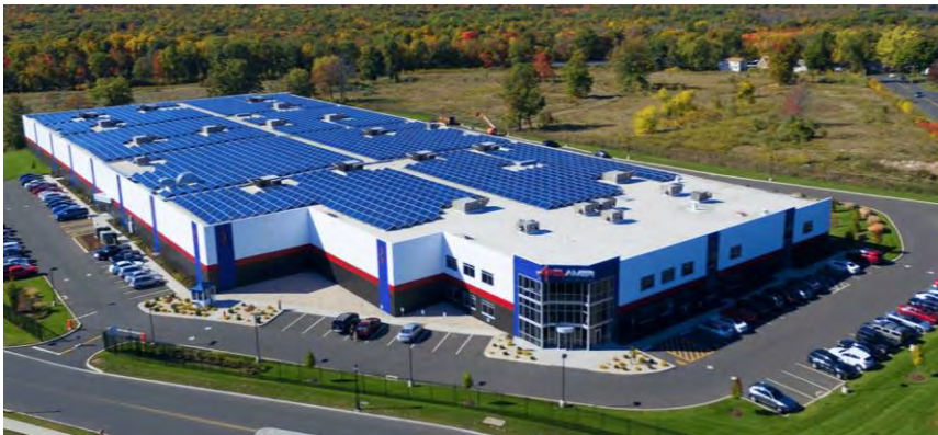
Polamer Precision, Inc.'s new 145,000 SF facility in New Britain sits on 8.3 acre site
