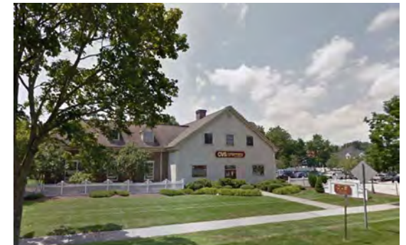
Pedestrian connection between the sidewalk and front entrance of a commercial building
